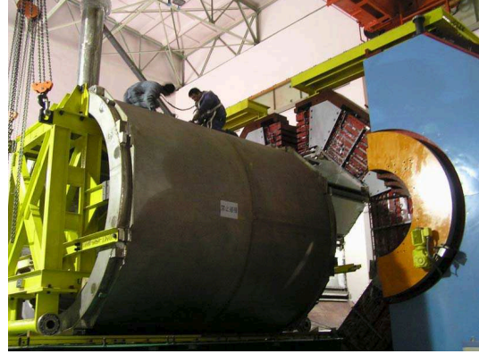
Figure 6. The super-conducting magnet during the installation into the BESIII detector. .
