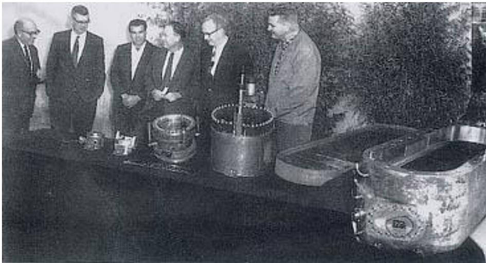
*Fig. 1. The 2", 4", 6", 10", 15" and 72" bubble chambers built at Berkeley, in the early days of the BC era.*
