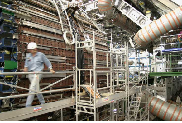
Figure 1: The ATLAS cavern in October 2005, insertion of the calorimetric systems. The coils of the ATLAS toroidal magnetic system are also visible.
