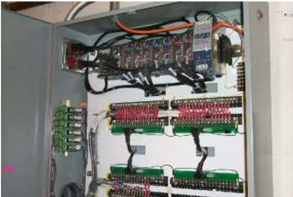
Figure 3: PLC in interlock chassis.
