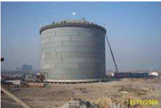
Figure 5. A typical 10 kton tanker for LNG storage.
