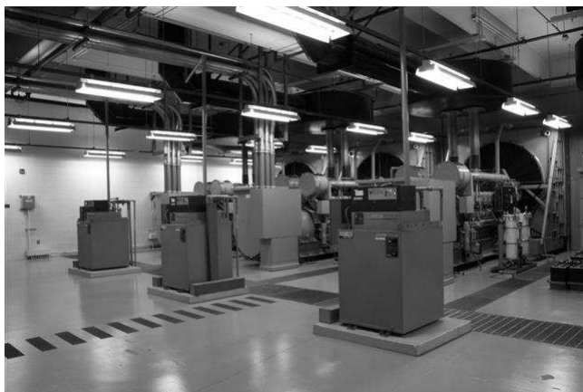
Figure 6: Microsoft Blue Ridge Generator Room
