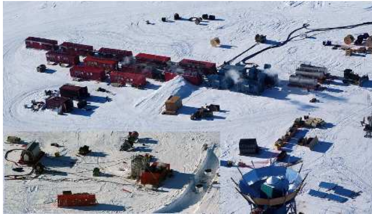
Figure 2. IceCube drill camp with drill tower image inset in lower left corner. The tower sits atop a drill hole. Two icetop tanks forming a station are visible in trench to the right of the drill tower.
