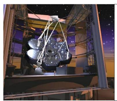
The GMT design. The telescope has 8m Magellan style segments, with relatively large gaps between the segments. The attraction is that the mirrors can be made with a proven technology and the problems of phasing are reduced. The secondary mirror is composed of a set of matched smaller mirrors which simplifies the control problems.
