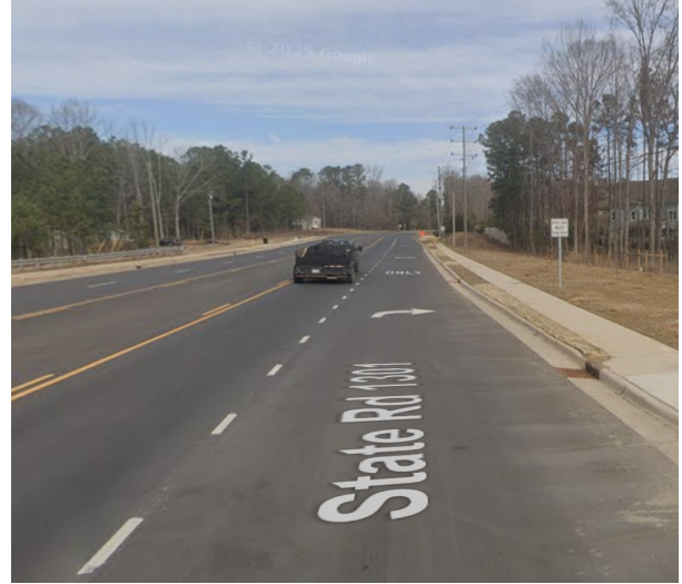
(b) Field view of the experimental roadway segment.
