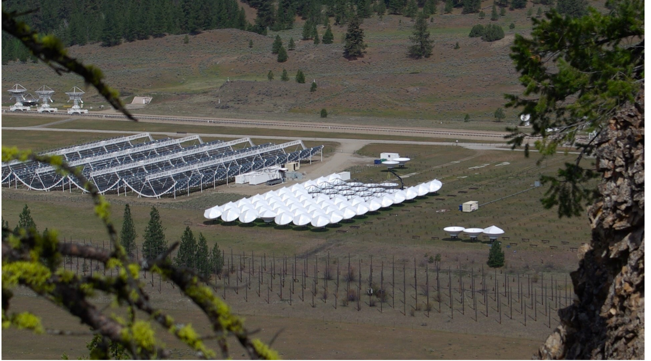
Figure 9. Photograph of the CHORD core array at the Dominion Radio Astrophysical Observatory on April 28, 2026, following installation of the 64th dish. Dishes with and without radomes are shown. At the time of writing, all 64 dishes of the initial pathfinder array had been installed on their completed foundations, with integration of the analog, digital, and networking systems underway in preparation for first-light commissioning observations. The remaining dishes of the 512-element core array are planned for staged deployment through 2027, with commissioning of the full instrument expected in 2028. Image by Brian Hoff
