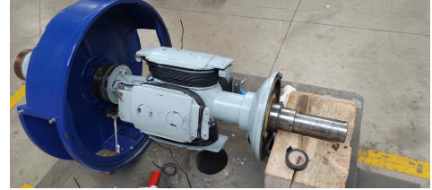
Fig. 6. Modification of the selected generator's field winding to allow external taps for controlled fault injection.
