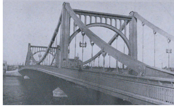
(b) Kiyosubashi Bridge
