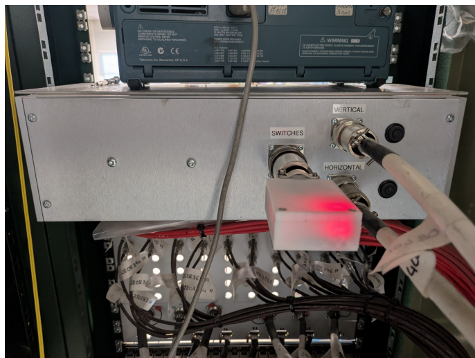
Figure 7: Rear view of the PS T9 DESY Table control panel with the NA64-DTC device installed.
