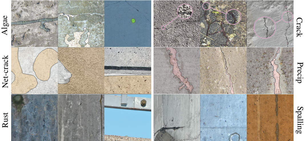
Figure 2: Mosaic of the six defect types in tiled images.
