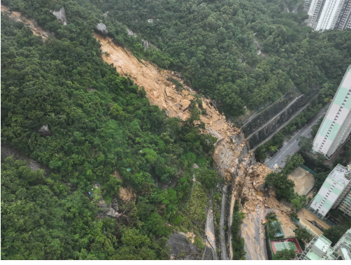
Figure 1. Severe landslide occurred at Yiu Hing Road, Shau Kei Wan, Hong Kong.
