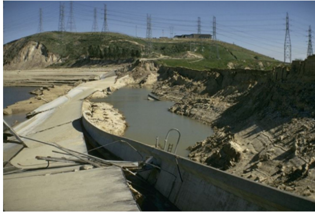
Figure A.1: Lower San Fernando dam failure (Chowdhury, 2018)
