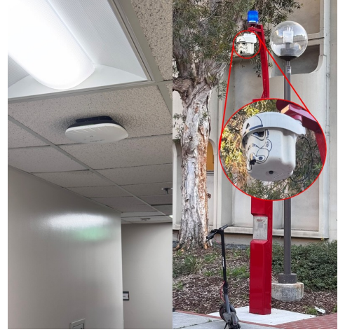
Fig. 4: Example photos of indoor (left) and outdoor (right) APs deployed across the campus.
