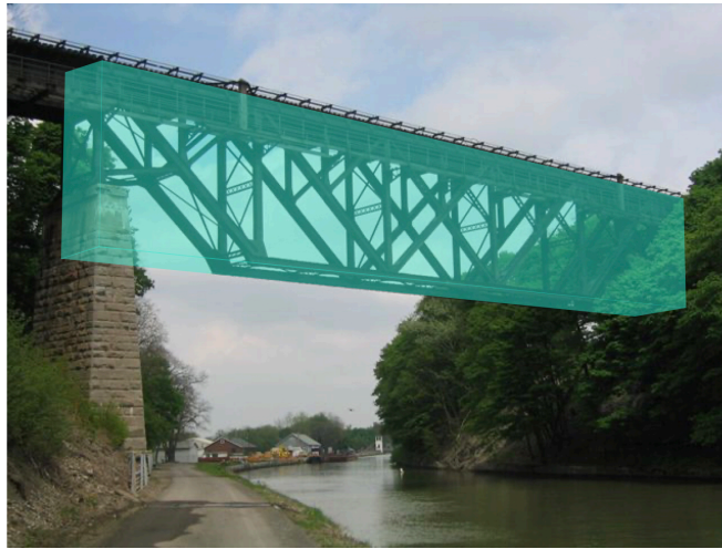
Figure 16: Lockport truss bridge passing over the Erie Canal near Buffalo, New York. The design space used in the following examples that aims to mimic this structure is highlighted in teal blue.
