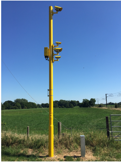
(a) Surveillance camera at level crossing
