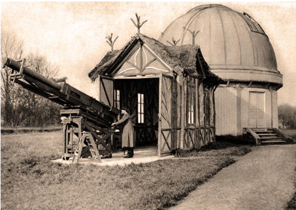
Figure 18 : Janssen's 135 mm/2.2 m refractor in the garden of Meudon, in 1880. OP Credit.
