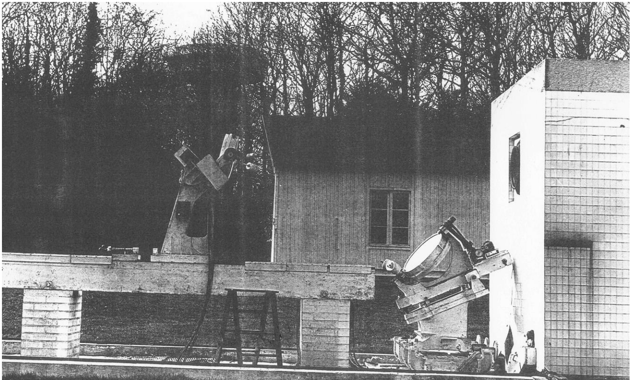
Figure 76 : coelostat with two plane mirrors which fed the 9 m spectrograph before transport to the Pic du Midi. In the background, the solar tower being finished in 1970. OP Credit.
