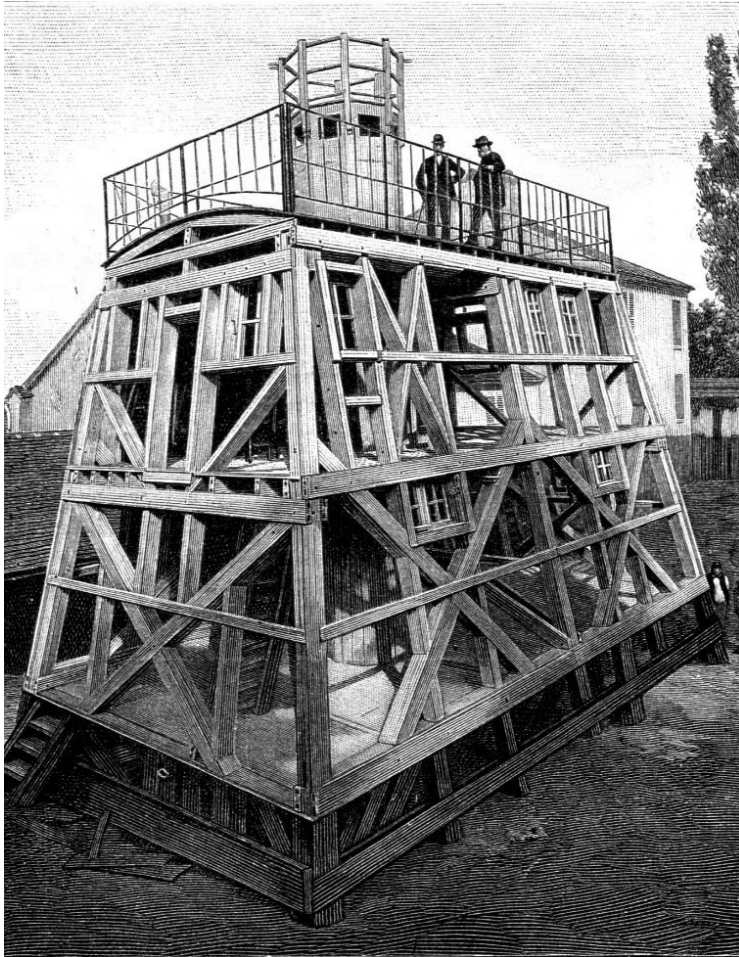
Figure 24 : the Mont Blanc observatory built and tested in Meudon before being transported on the back of carriers or by sleigh to the summit. On the right, the small spectrograph of 1 m. Credit OP.
