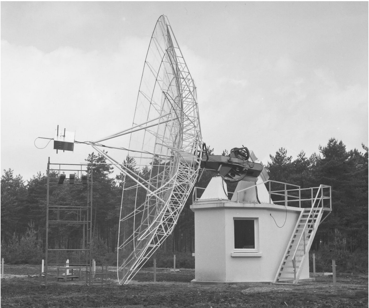
Figure 104 : additional large antenna of 10 m from the Nançay radioheliograph. OP credit.
