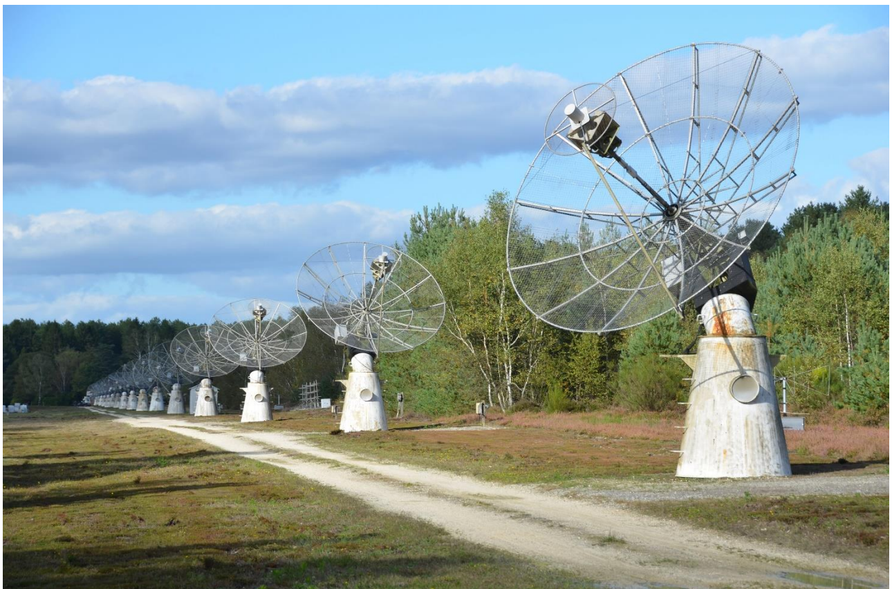
Figure 103 : metric radiotelescope (150 to 450 MHz) of Nançay, with two orthogonal kilometre-length baselines totalling about 50 antennas. Credit OP.
