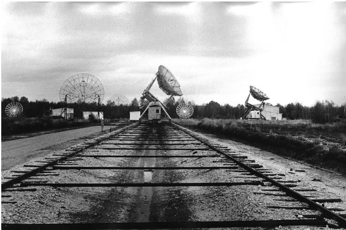
Figure 99 : the two Würzburg radars installed in Nançay in 1953 on rails, allowing to change their respective distance and develop interferometry. OP Credit.
