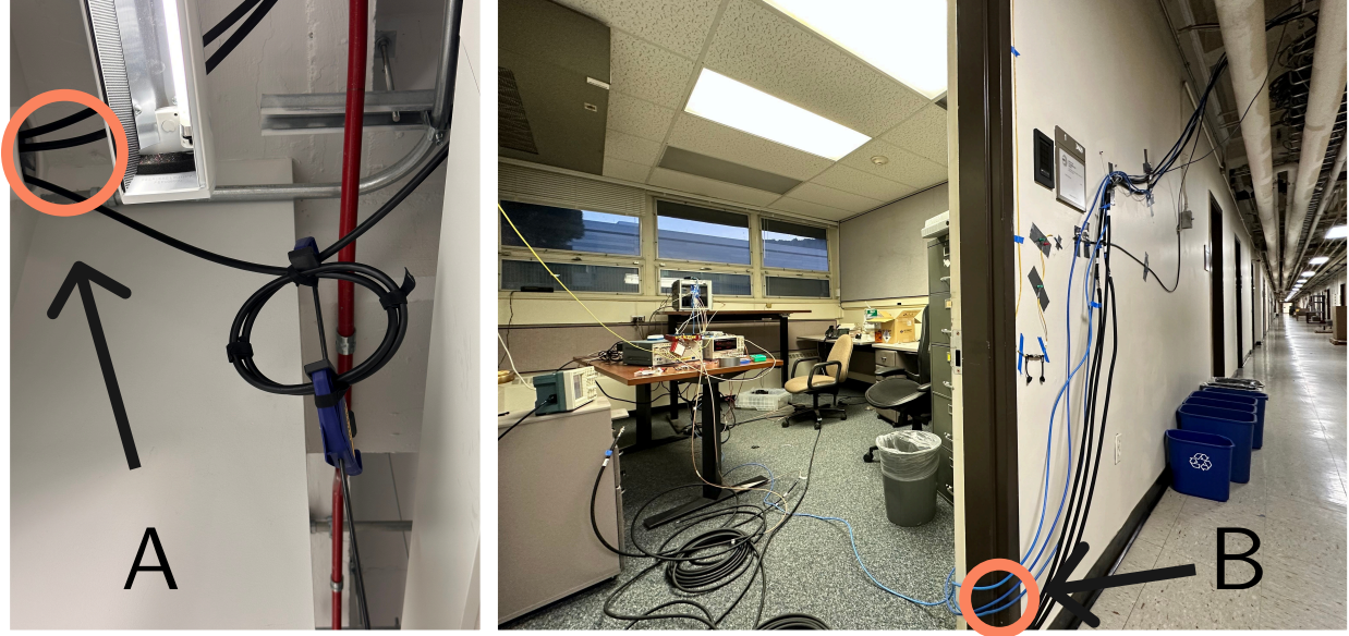
FIG. 6. Photographs of the physical entry/exit points of the classical and quantum signals that serve as the verifiers A and B in our demonstration. Any hardware and cabling inside the verifier labs is trusted. At verifier B, the lab houses a random number generator for deciding the challenge u_B , and a timetagger that records classical timing information and the response from provers z_B . All information exiting and entering the Verifier B lab is classical.
