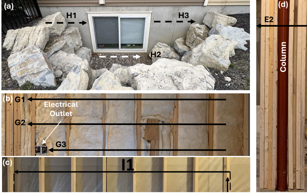
Figure 2: Each wall in the dataset is assigned an alphabetic label, and individual wall segments are indexed numerically; the resulting alphanumeric identifier uniquely specifies each GPR scan. Panel (a) shows exterior wall segments with partial rock background (H1 and H3) and soil background (H2). Panel (b) shows interior wall segments, including G1, as well as G2 and G3, which are located near electrical outlets. Panel (c) shows an exterior wall segment (I1). Panel (d) shows an interior wall segment (E2) containing an embedded column. Unless otherwise noted, wall segments I1 (exterior) and G3 (interior) are used in the training set for all classification and interpretability tasks considered in this study, with the exception of the wall-background classification task.
