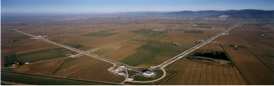
FIG. 10: The Virgo Observatory in Santo Stefano a Macerata, near Pisa, Italy. It is part of the European Gravitational Observatory. Viaducts were built above each of the 3 Km arms to allow vehicles from neighboring farms to pass.
