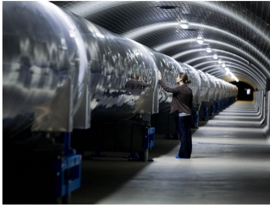
FIG. 11: Gigantic vacuum tube housing the lasers along the 3 km arms of the Virgo Observatory.
