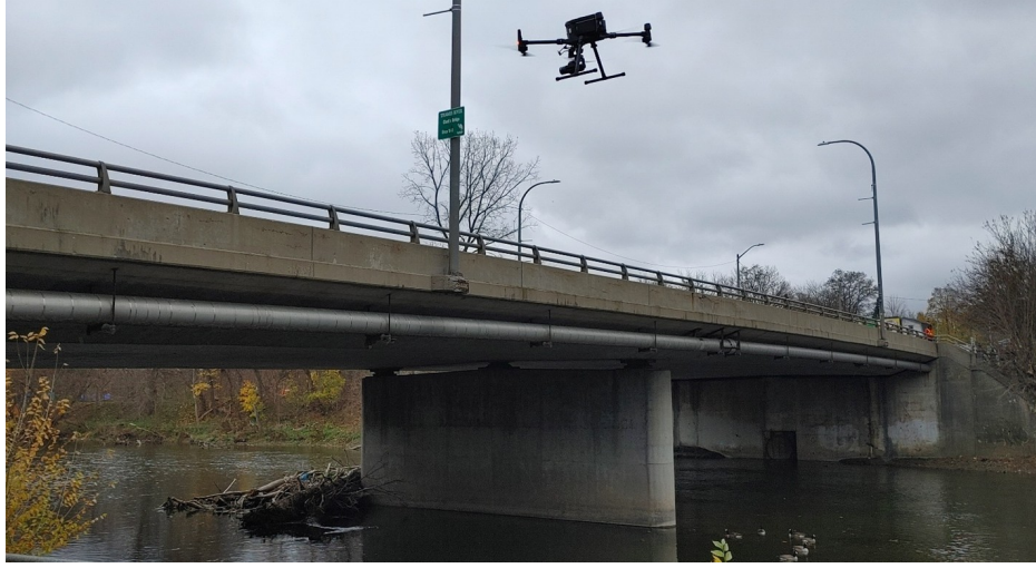
Figure 13: Full-scale city bridge inspected using a lidar and camera-mounted drone.
