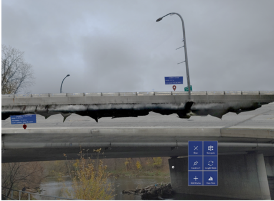
Figure 14: 3D model projection of the bridge on the real structure.
