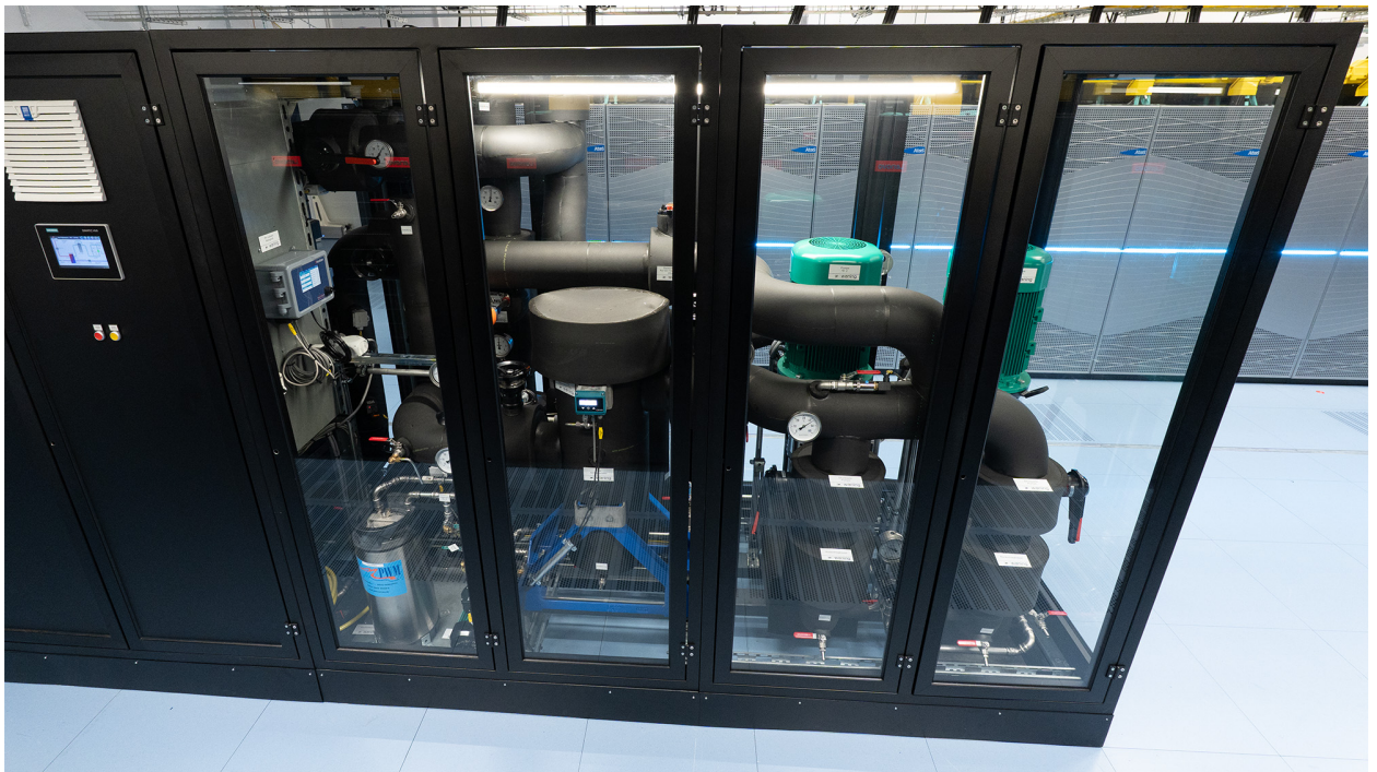
Figure 19: Central Cooling distribution unit of OTUS supercomputer. All connecting pipes are located below the raised floor.
