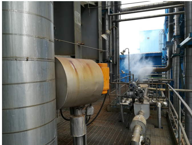
Figure 2: The desuperheater (DSH) unit at the Pareh-Sar power plant, where valve leakage has been identified as a critical fault source affecting steam temperature regulation.
