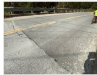
Deck & upstream rail from abutment 1
