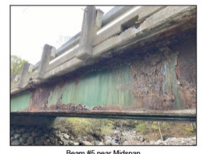
Beam #5 near Midspan
