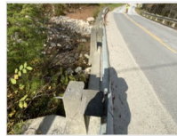
Upstream rail from abutment 1
