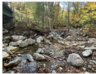
Upstream of abutment 1
