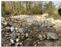
Upstream of abutment 2
