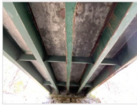
Deck & superstructure abutment 2
