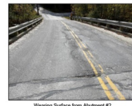
Wearing Surface on Abutment #2
