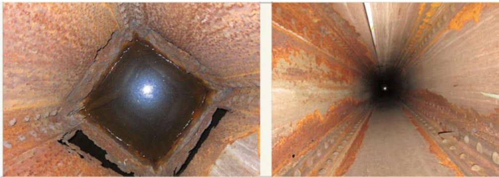
Figure 1 Inside Column Showing Water and Large Holes Caused by Rusting
