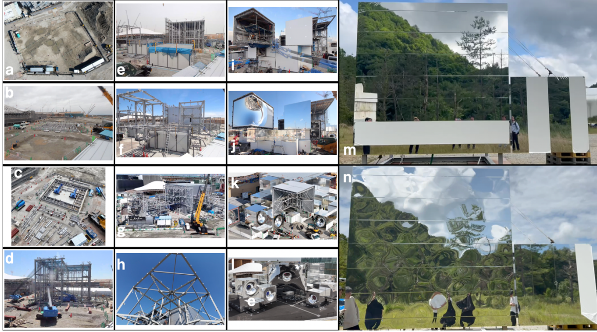
Figure 4. Construction process of the null 2 pavilion. (A) Cleared and segmented site. (B) Theater foundation construction begins. (C) Theater foundation completed, starting building construction. (D) Theater steel framework assembled. (E) Completion of theater framework, installation of prefab units for management and security buildings. (F) Facade structural assembly initiated. (G) Facade structure nearing completion. (H) Main facade structure completed. (I) Mirror membrane installation begins. (J) Quality check of installed mirror membrane. (K) Mirror membrane installation nearly complete. (L) Pavilion fully completed. (M) Outdoor weather durability test of mirror membrane. (N) Vibration testing of mirror membrane.
