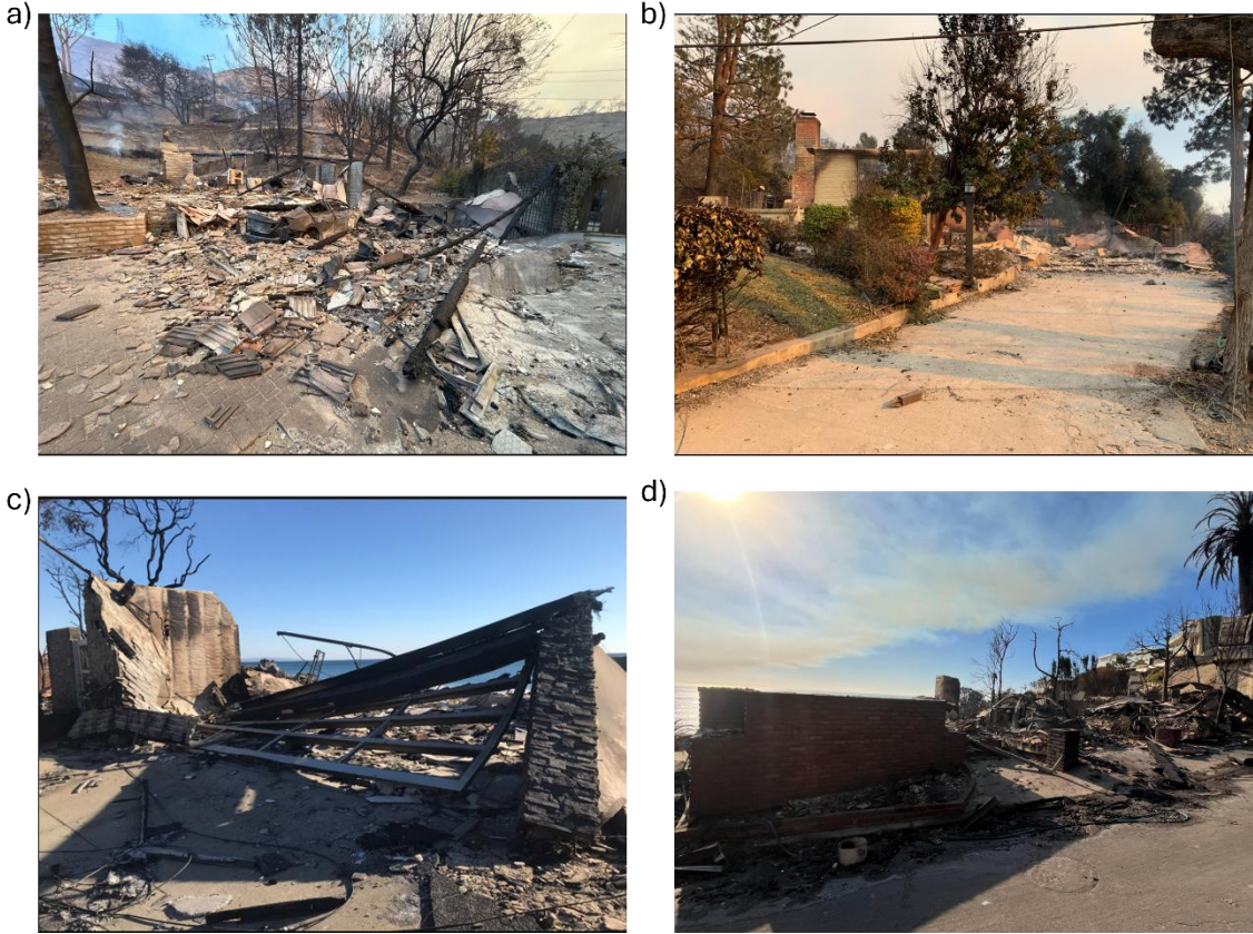
Figure 9. Cases in which both single view and multi-view were classified correctly in Pipeline b. Figure 6 (a–d) were classified as destroyed in ground truth labeling. All homes in this figure only had one single view. Figure 6(a) and (b) are in Eaton; Figure 6 (c) and (d) are in Palisades.
