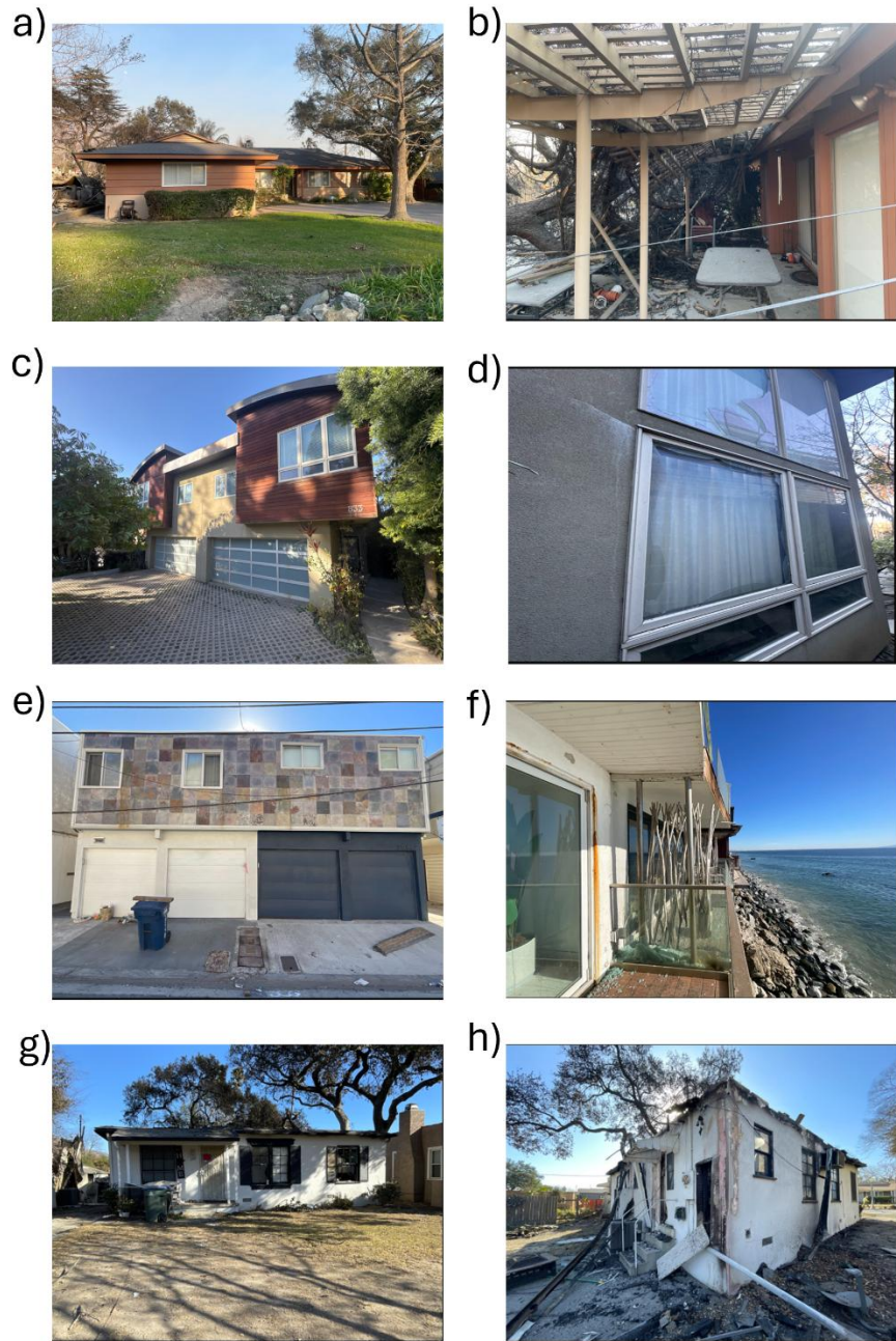
Figure 10. In each row are pairs of images for the same house; front views of houses ((a), (c), (e), (g)) were classified as no damage. In the multi-view assessment, (a)–(b); (c)–(d); (e)–(f); and (g), (h) were inputs for the Pipeline B. They were classified as affected which matches the ground truth label.
