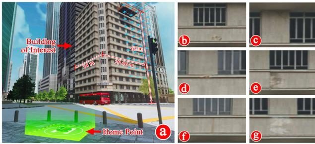
**Figure 3: The simulated building inspection scenario and different types of defects used in our study. (a) Overall configuration of the scenario. (b) Paint peel. (c) Wall crack. (d) Wall dent. (e) Rotten surface. (f) Leakage. (g) Delamination.**
