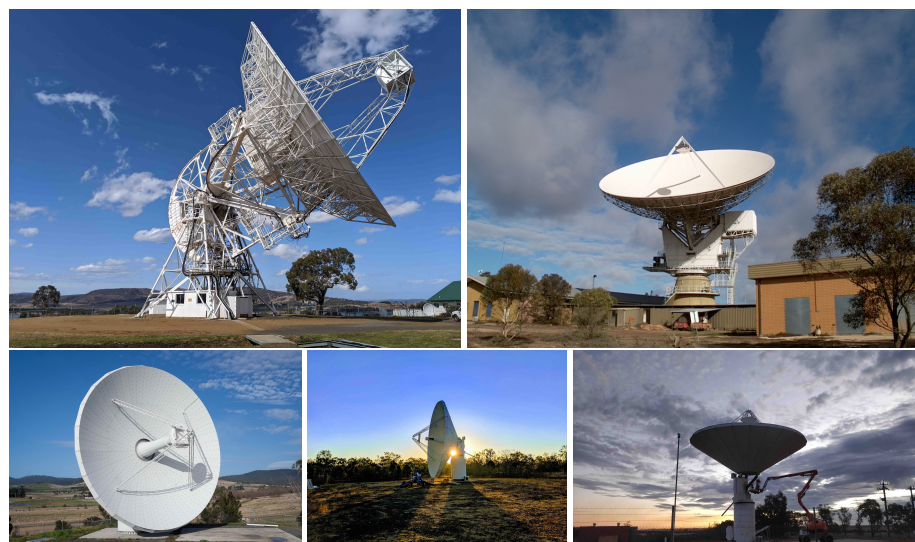
Figure 1. UTAS radio telescopes. From top left in reading order are the Hobart 26 m, Ceduna 30 m, and the Hobart, Katherine and Yarragadee 12 m antennas.
