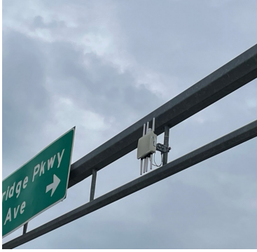
(a) RSU installed at the intersection.
