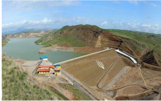
Figure 1 A view of the dam's body, the lake, and the exploitation buildings(46)
