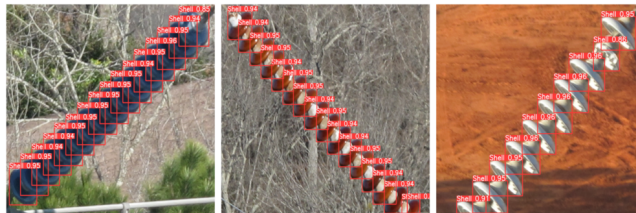
Fig. 3: Detection results on a sample of shells from the test dataset. One can see that shells are detected in a variety of environments, orientations and colors.
