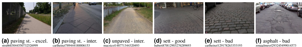
Figure 1. Example images of different surface types and qualities, with Mapillary contributor names and image IDs.
