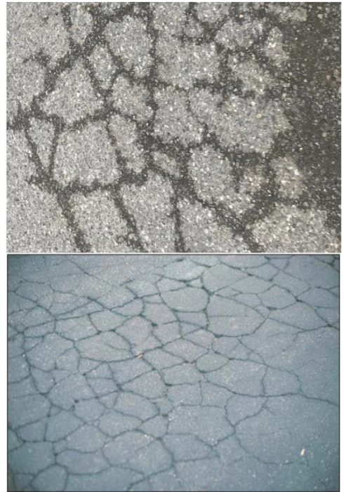
Fig. 5. High Severity Fatigue Cracking.
