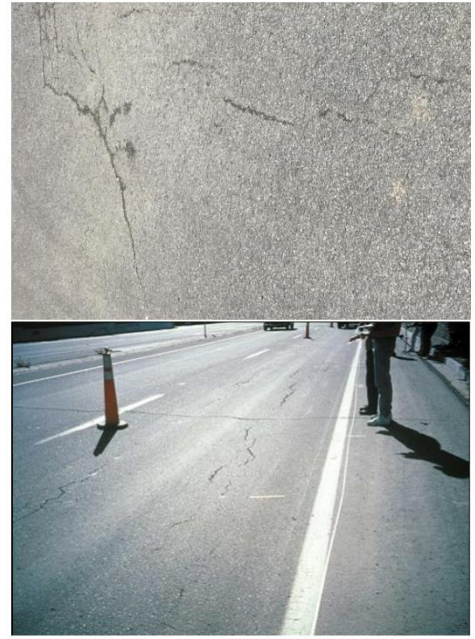
Fig. 4. Low Severity Fatigue Cracking.
