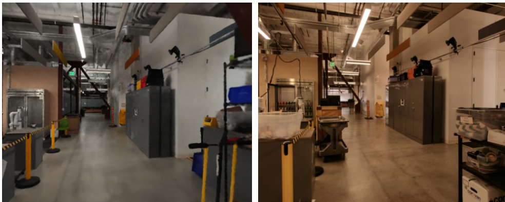
(a) NeRF render of the simulated Office environment (b) Real image of the Office environment
