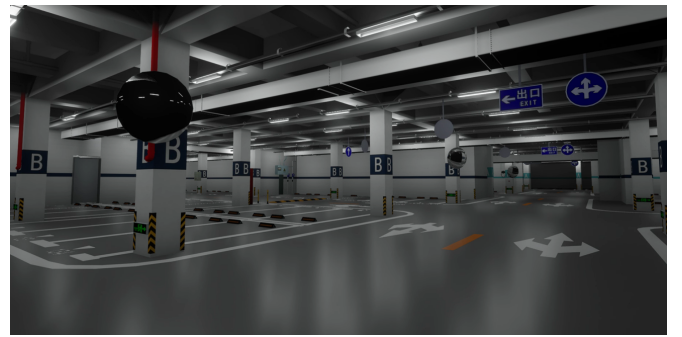
Fig. 1: Carla simulation environment of the underground parking garage. The model is a 1:1 simulation of the underground parking garage at the Southern University of Science and Technology of Engineering, including lane markings, parking spaces, and traffic signs with semantic information.
