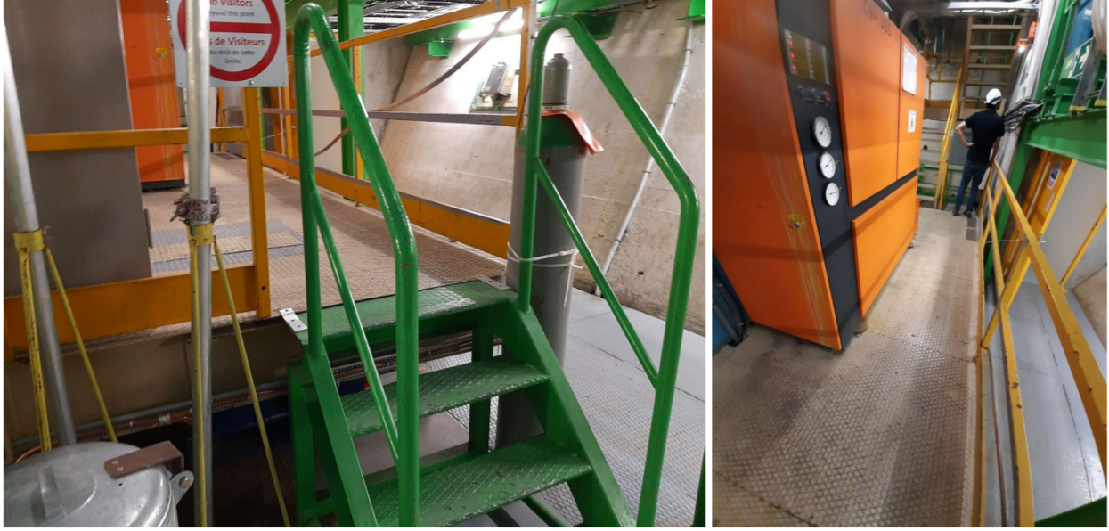
FIG. 17. Pictures of the entrance to the D1 barracks, showing the staircase and gangway, and corresponding to the highlighted area with a blue rectangle in Figure 16.
