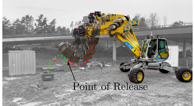
Fig. 1. Two-dimensional throwing controller deployed on the M545 excavator with overlaid payload trajectory.
