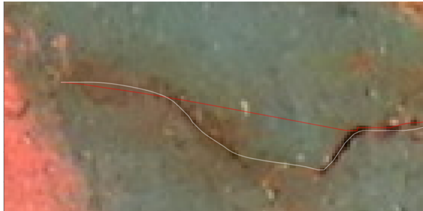
Fig. 3: Close up view of a crack with their calculated crack path retrieved by two methods: The red line shows the track obtained by tracking in \mathbb{R}^2 while the white line shows the spatially projected track obtained by tracking in \mathbb{M}_2 = \mathbb{R}^2 \times S^1 .
