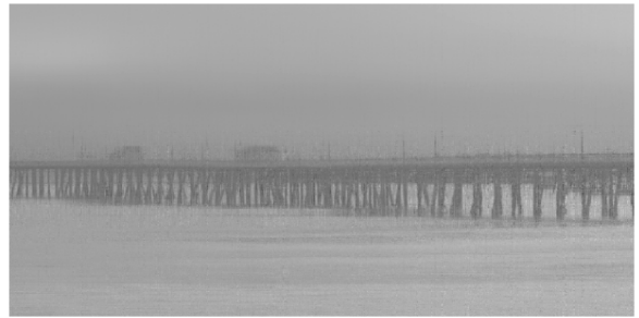
Bridge restored with CSNN-0.5
