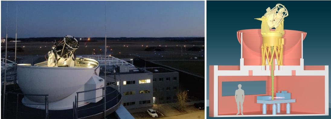
**FIGURE 1** The OGSOP-new 80 cm Ritchey-Chretien Telescope, and adjacent functional Diagram of OGSOP-new with Coude-Room underneath hosting various experiments for AO and QKD. Image: DLR
