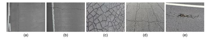
Fig. 2. Example snapshots of various types of road surface defects: (a) Transverse crack, (b) Longitudinal track, (c) Alligator crack, (d) Block crack, and (e) Pothole. It is important to note that T the key difference between (a) and (b) is the angle with the road lane. If the crack runs parallel to the road lane, it is classified as a transverse crack. Conversely, if the crack is at a right angle to the lane, it is classified as a longitudinal crack.
