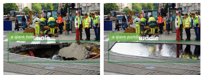
Positive: A bunch of people are standing on a street that has a giant hole in it Negative: A bunch of people are standing on a street that has a giant puddle in it
