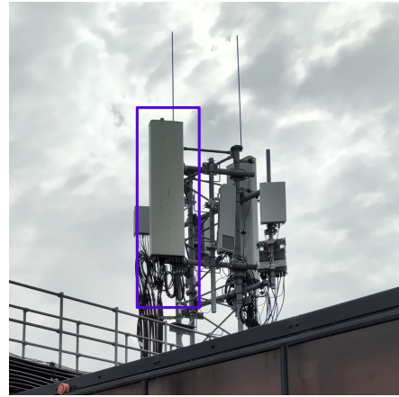
Fig. 5. Sector antenna used in the measurements. The main lobe is directed north, with 90^\circ and 6.5^\circ beamwidths in azimuth and elevation, respectively.
