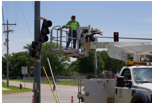
Caption: A worker takes a stoplight down from the pole.
