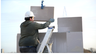
Fig. 1: Laying of a suspended block.
