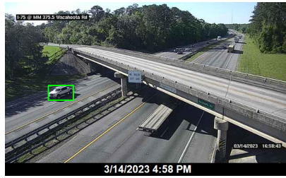
(b) Bridge obstructs view on highway, cars passing over the bridge occasionally in a third direction
